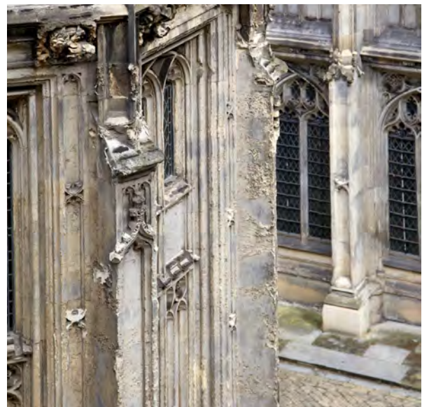
Figure 6. The effect of exposure to elements on stonework can be seen in Cloister Court.
